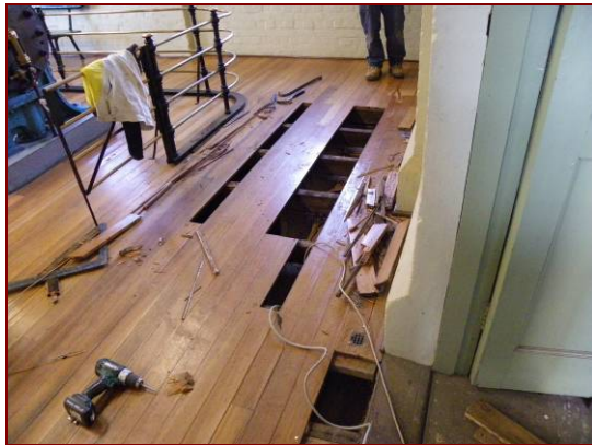
Figure 4.69: Replacement of rotted floorboards in southern annex, above pumpwell.
