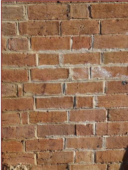
Figure 4.75: Replaced mortar where it had previously failed.
