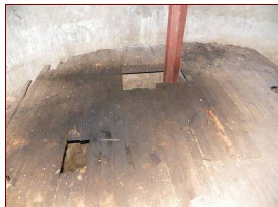
Figure 4.68: Damp, rot and degradation of timber floorboards on first level of pump well.
