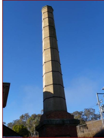
Figure 4.17: Chimney stack showing iron clamps.
