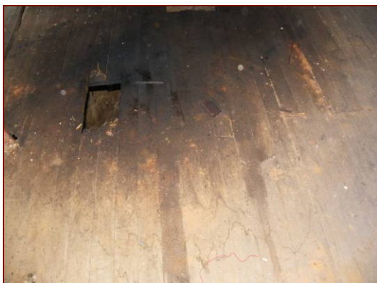
Figure 4.67: Damp, rot and degradation of timber floorboards on first level of pump well.
