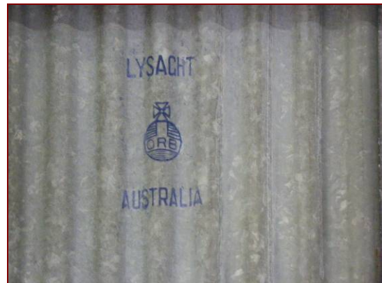
Figure 4.35: Lysaghts orb on the underside of the roof material in the southern Annex.
