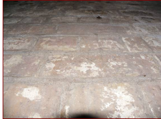
Figure 4.72: Small amounts of failing limewash and salt on walls within subfloor area.
