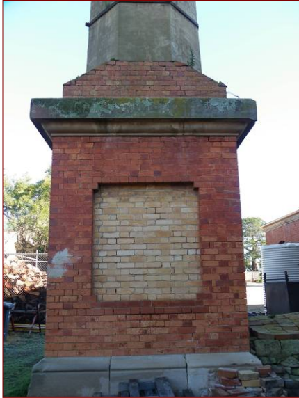
Figure 4.16: Chimney stack base with contrasting brick work plus sandstone base and corbel.
