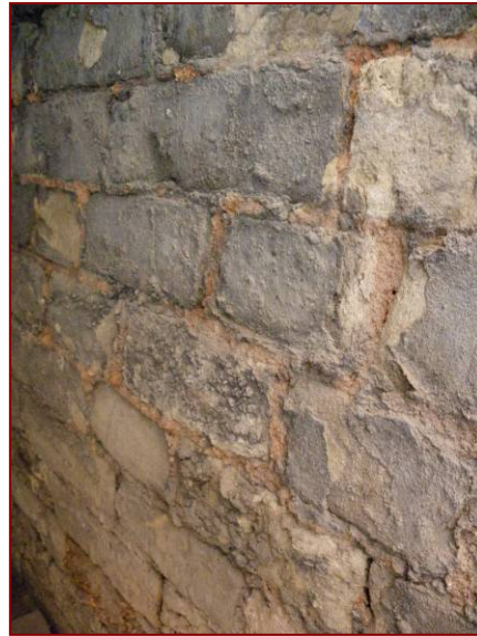
Figure 4.58: Salt attack and brick delamination in the tunnel.
