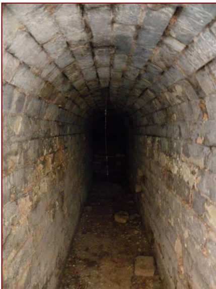
Figure 4.46: Interior tunnel from the Boiler Room to the chimney stack.
