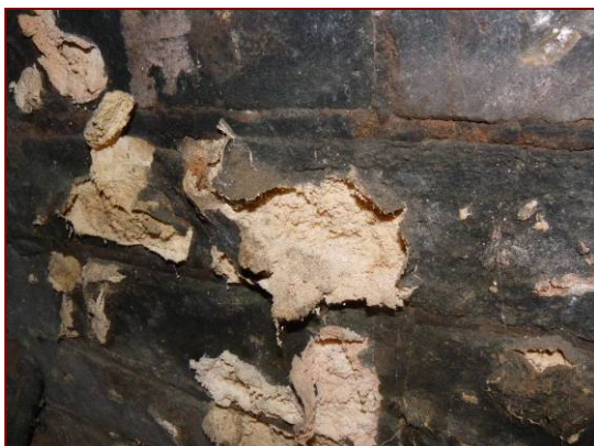
Figure 4.61: Severe and advanced salt attack within the chimney, resulting in delamination of the bricks.
