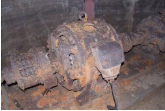
Figure 4.104: Crompton Motors with severe active rust.
