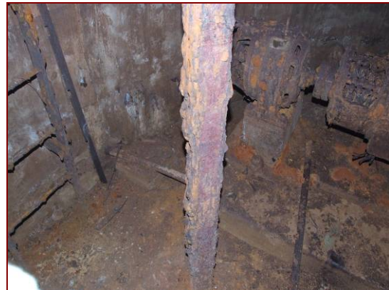
Figure 4.66: Severe rust and corrosion on lower floor of pump well affecting steel supports and pumping equipment (Image courtesy of Ian McCormack).
