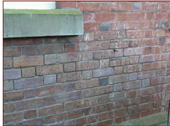
Figure 4.84: Failed mortar, algae growth and the beginnings of salt attack, southern elevation.
