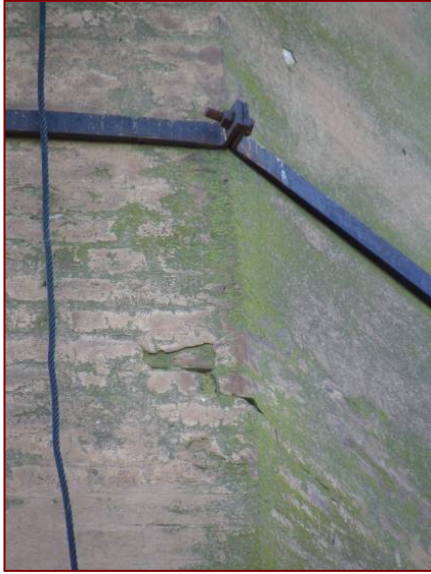
Figure 4.53: Algae growth and cracking of render on the chimney stack.
