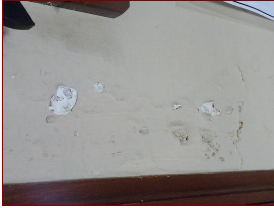
Figure 4.71: Bubbling paint on wall above staircase leading down to the sub-floor area.
