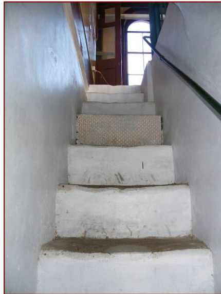
Figure 4.72: Small amounts of failing limewash and salt on walls within subfloor area.
