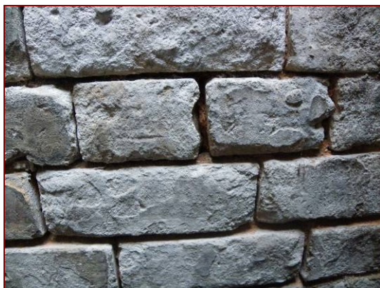
Figure 4.55: Almost complete loss of mortar within the tunnel.
