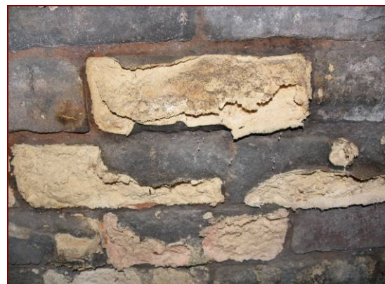
Figure 4.62: Severe and advanced salt attack within the chimney, resulting in delamination of the bricks.
