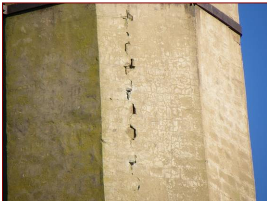
Figure 4.49: Cracking of the render on the upper areas of the chimney.
