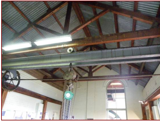
Figure 4.44: Northern annexes timber trusses and overhead crane.
