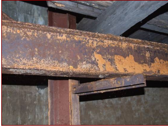
Figure 4.63: Corrosion of steel girders within southern annex pump well (Image courtesy of Ian McCormack).
