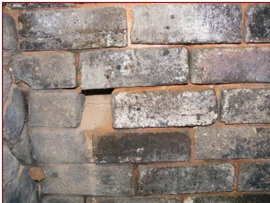
Figure 4.59: Almost complete loss of mortar and salt attack within the base of the chimney.
