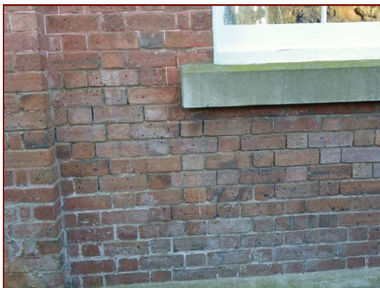
Figure 4.85: Failed mortar, inappropriate concrete mortar and the beginnings of salt attack, southern elevation.
