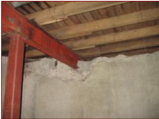
Figure 4.65: Degradation of concrete where steel girder is in contact with the concrete pump well (Image courtesy of Ian McCormack).
