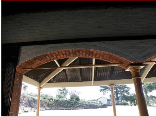
Figure 4.18: Brick arches to western elevation of the Boiler Room.
