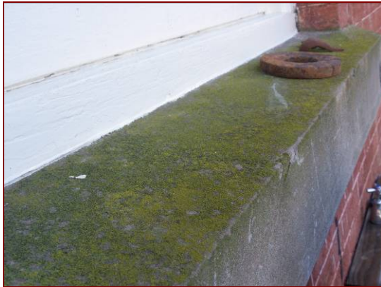
Figure 4.83: Algae on sandstone window sill, south elevation Boiler Room.
