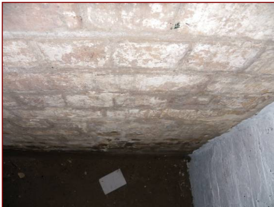
Figure 4.73: Small amounts of failing limewash and salt on walls within subfloor area, plus mildew on base of wall.
