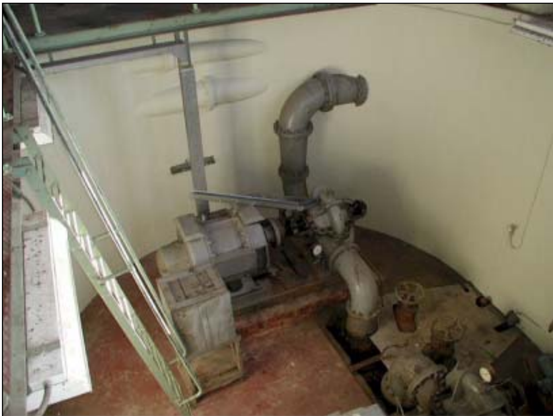
Electric Pumps in well – East Annex
