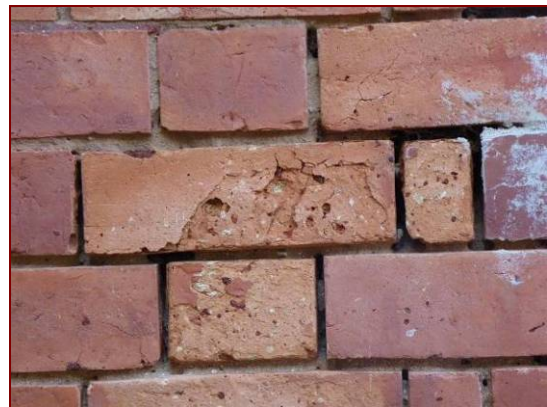
Figure 4.50: Loss of mortar and delamination of bricks on chimney base.
