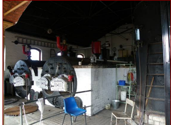
Figure 4.19: Interior of the Boiler Room looking north-east showing horizontal boilers.
