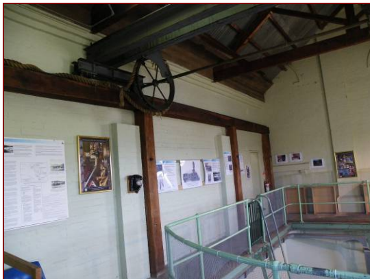
Figure 4.42: Northern Annex showing timber support system for the overhead crane.
