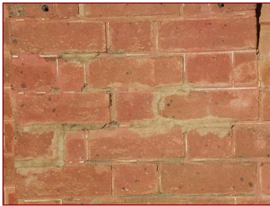
Figure 4.79: Failed mortar replaced inappropriately with concrete mortar – north elevation.
