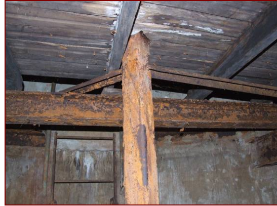
Figure 4.64: Corrosion of steel girders, rot in floor board underside and evidence of salt on concrete walls in pump well (Image courtesy of Ian McCormack)..
