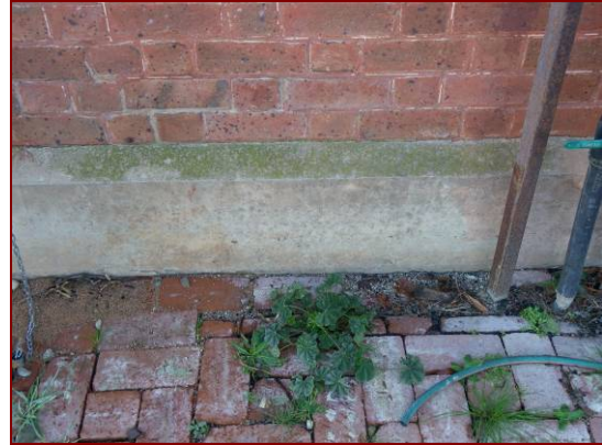
Figure 4.82: Algae growth, southern elevation.
