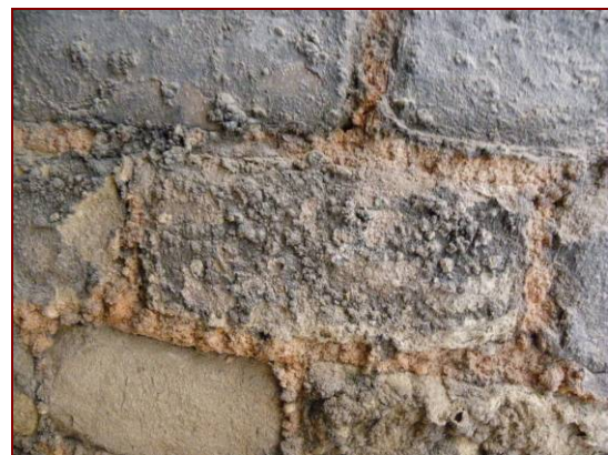
Figure 4.56: Advanced salt attack on the bricks and mortar, in the tunnel.
