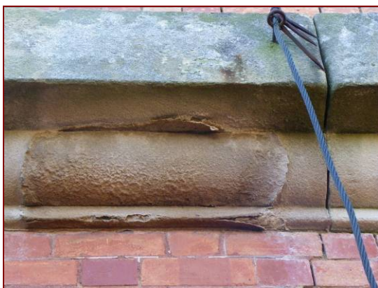
Figure 4.51: Algae, salt attack and delamination of sandstone.
