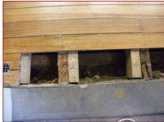
Figure 4.70: Replacement of rotted floorboards in southern annex, above pumpwell.
