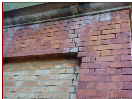
Figure 4.52: Algae, salt attack and loss of mortar.
