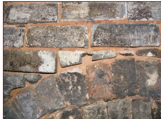
Figure 4.60: Loss of mortar and the beginnings of salt attack (white patches) within the base of the chimney.
