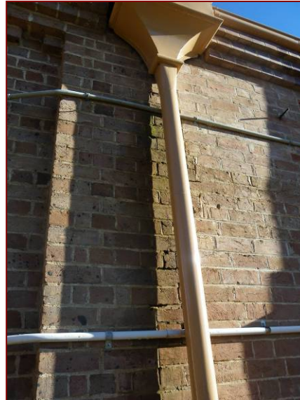
Figure 4.76: Damp and algae behind failing downpipe.
