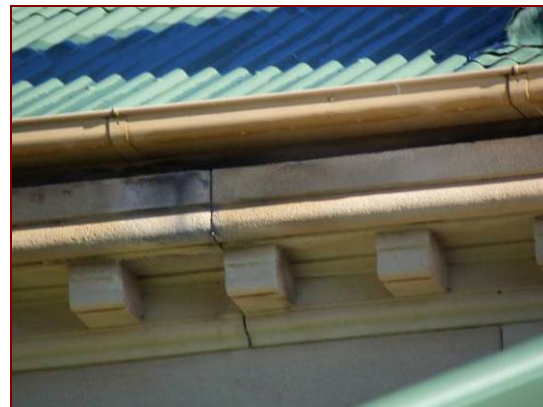
Figure 4.78: Damp causing mildew and mould to sandstone corbels underneath a failing downpipe.
