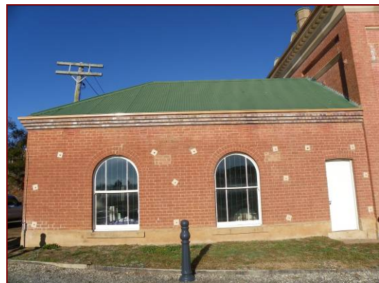
Figure 4.86: Raised garden beds against northern wall of the Northern Annex – this will be contributing to the damp problems.
