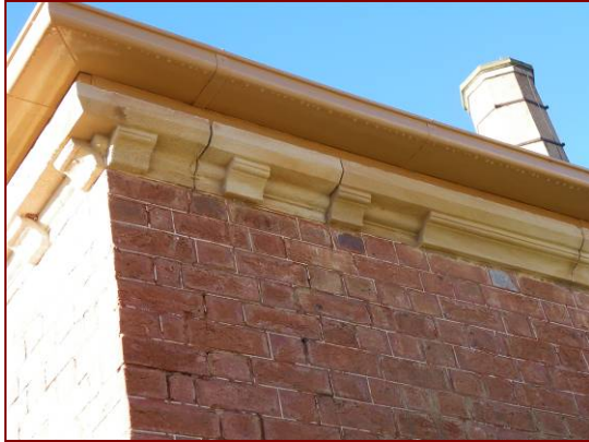
Figure 4.81: Failed mortar and cracking, upper north-west corner of Pumphouse building.
